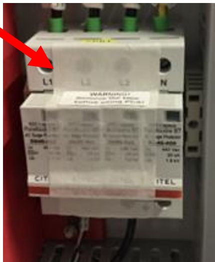
Figure 49. Remove the adhesive tape on AC SPD
