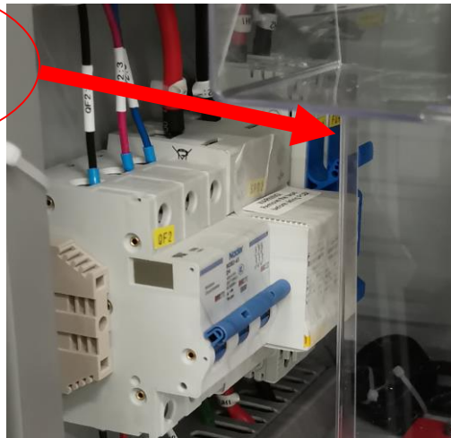
Figure 48. Remove the adhesive tape on DC SPD
