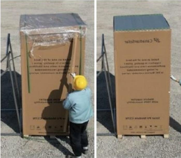
Remove the paper beams at the corners of the pallet, and then use the paper beam to remove the top cover and plastic wrap.
