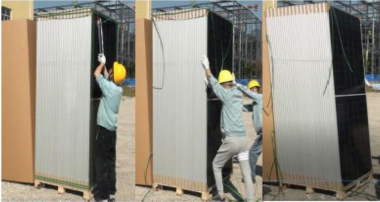
First cut the horizontal inner ribbons and keep the internal tapes vertical.
