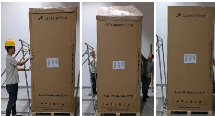
Remove the outside paper beams
