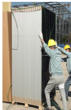
Cut 4 vertical straps and push modules to the rack
